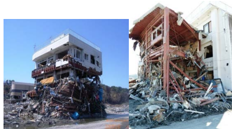
Fig. 1 Debris impact on structures following the 2011 Tohoku Japan Tsunami (Nistor, 2011).
