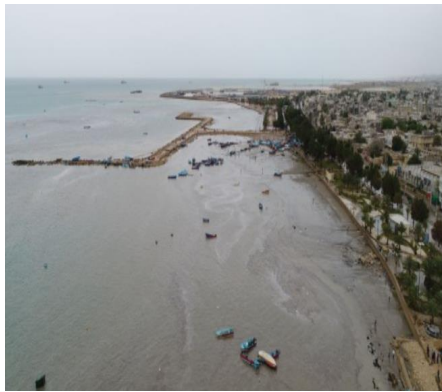
Figure 3. Dayyer port a day after storm incident.
