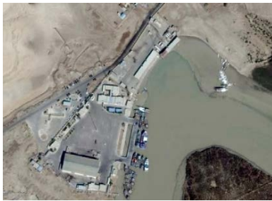
Figure 1. Aerial view of Sajafi Port
