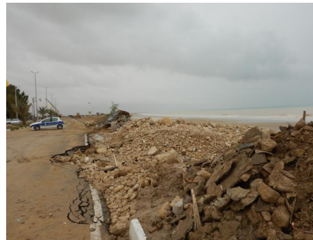
Figure 2. Photo of storm destruction
