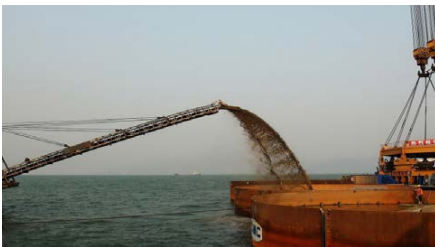
Figure 6. Filling the cylinders interior with sea bed sediments by using dredging ships.
