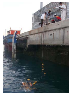
Figure 2. ROV Inspection of quay wall after receiving FBGs notification in Shahid Rajaei harbour
