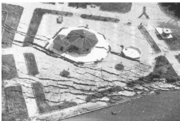
Figure 1. Liquefaction induced lateral spreading case after 1999 Kocaeli Earthquake.
