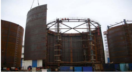
Figure 3. Cylinders under construction in shipbuilding and offshore industries.
