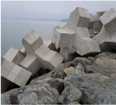
Figure 3. Photo of the xblocs on the filter layer from the project site
