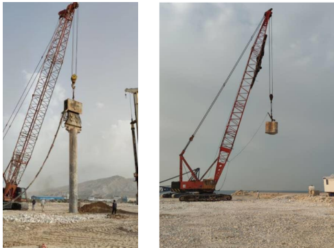
Figure 3. Implementation of dynamic replacement and stone column at the project site
