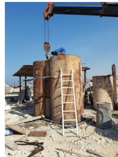
Figure 5. Special tampers used in project
