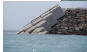
Figure 2. Xbloc and Cube armours in breakwater
