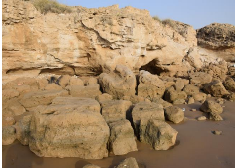
Figure 1. Severe coastal erosion of rocky shorelines of Genaveh city
