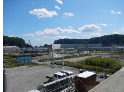
Figure 1. Case of Taro (High Embankment).
