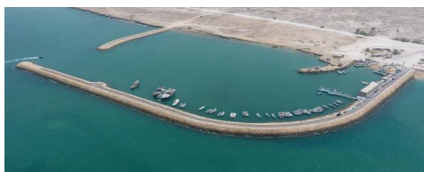
Figure 2. Kandaloo small breakwater
