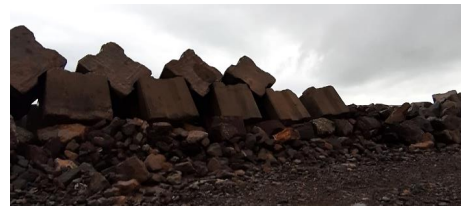
Figure 3. Placement method of antifer armour units (photo: January 2021, 21 st ).
