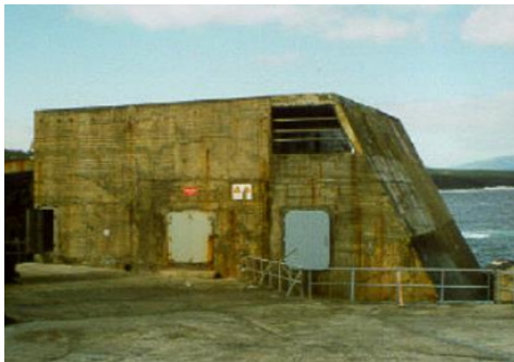
Figure 1. OWC structure
