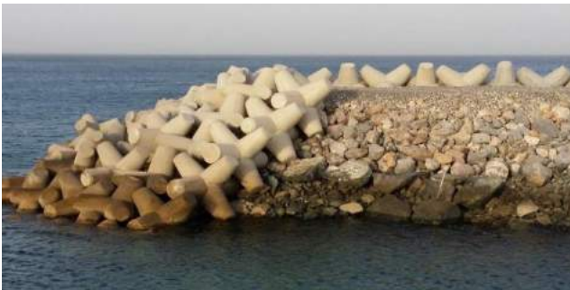
Figure 1. Crablocks as rubble mound breakwaters.
