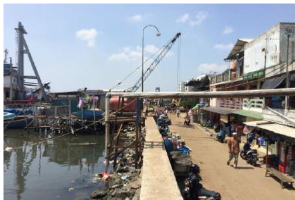
Figure 1. Thin concrete dyke protecting the Pluit District in Jakarta. Photo was taken at low tide, showing how water is already above the ground level in the district. (Photo: May 13, 2016).
