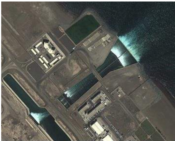
Figure 1. Areal view of the outfall at SIPA.
