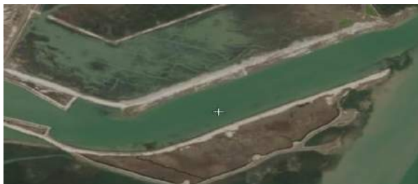
Figure5: After construction that inlets have been destroyed
