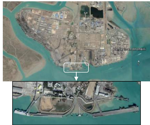
Figure 1. Location of under investigated coastal structures in Bandar Imam Khomeini (BIK) zone.
